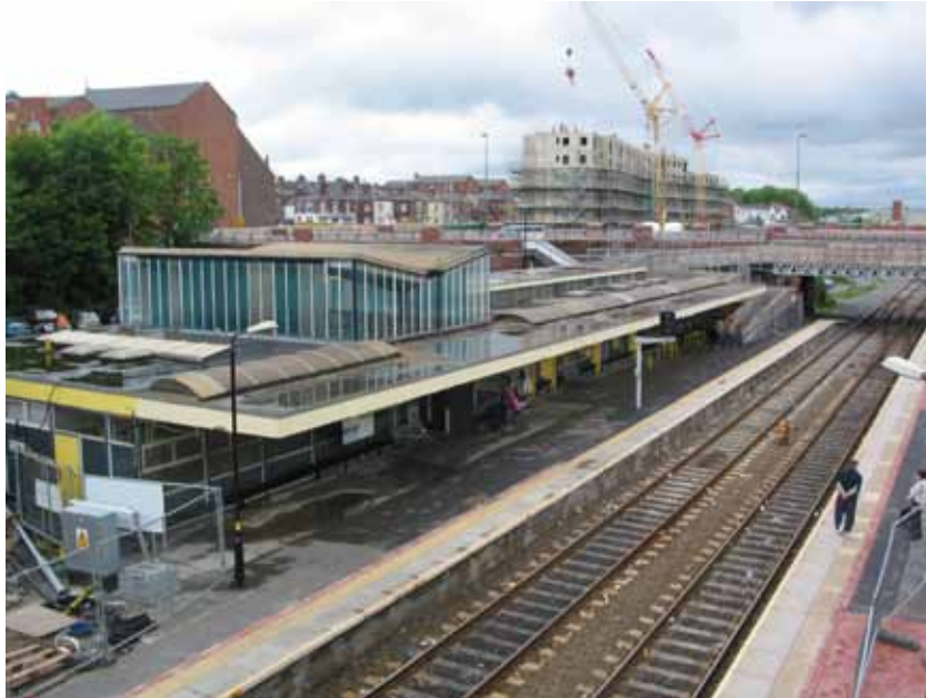
FIGURE 4.1 ST HELENS STATION BEFORE THE REDEVELOPMENT
