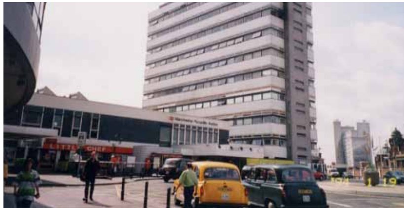
FIGURE 2.1 MAIN ENTRANCE TO MANCHESTER PICCADILLY (PRE-2002)
