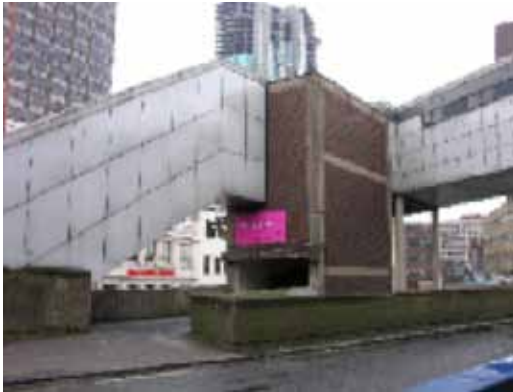
FIGURE 3.1 STATION STREET EXIT SOUTH OF BIRMINGHAM NEW STREET STATION
