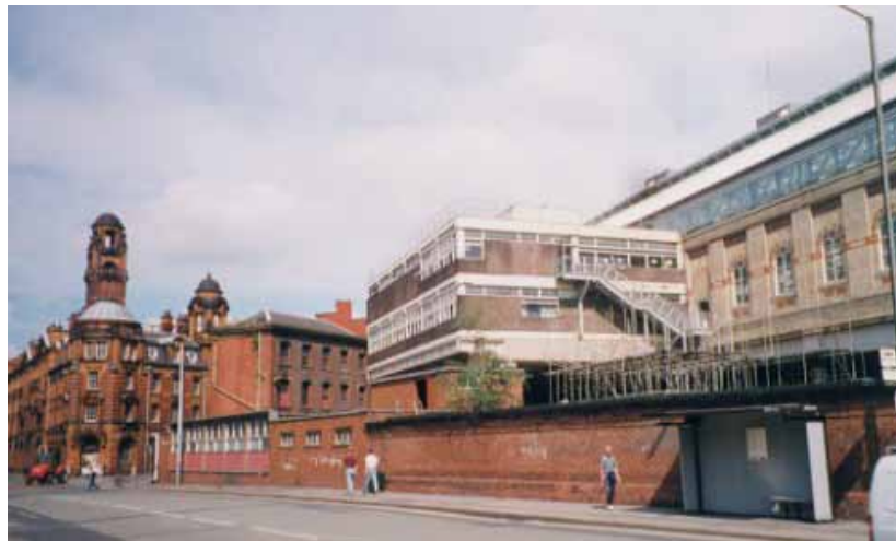
FIGURE 2.3 EXAMPLE OF RESTRICTED PHYSICAL ACCESS – MANCHESTER PICCADILLY C. 1994
