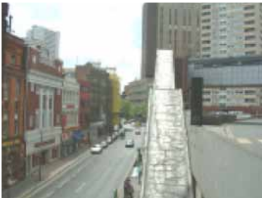
FIGURE 3.2 NEW STREET STATION HEADING SOUTH
