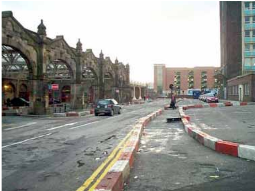
FIGURE 1.1 SHEFFIELD STATION & CAR PARK BEFORE THE INVESTMENT
