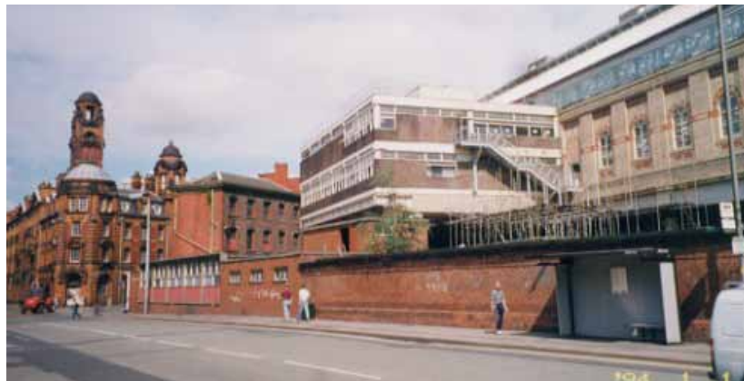
FIGURE 2.2 ENTRANCE TO MANCHESTER PICCADILLY FROM FAIRFIELD STREET (PRE-2002)
